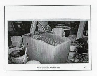
Wood burner must meet clearance to combustibles requirements & be labeled for use in a garage....
